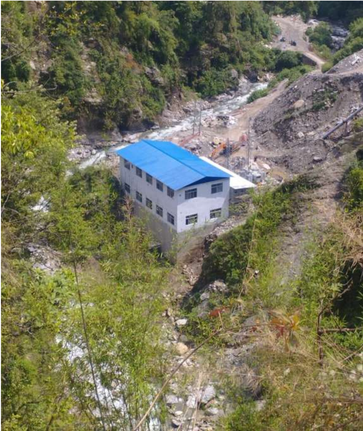
Photo 8-2 Powerhouse, control room and Switchyard
