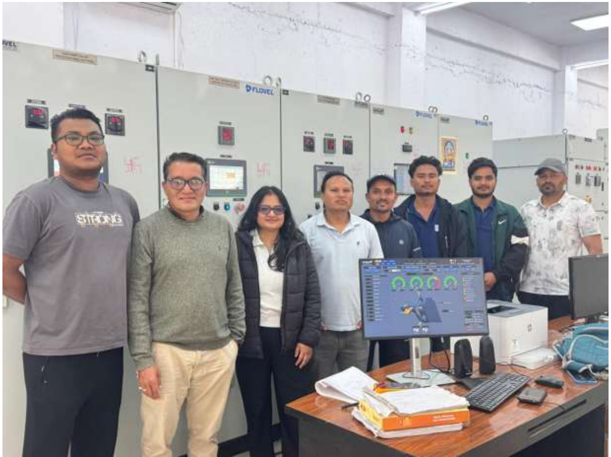
Photo 8-7 Successful Testing and Commissioning by NEA team members
